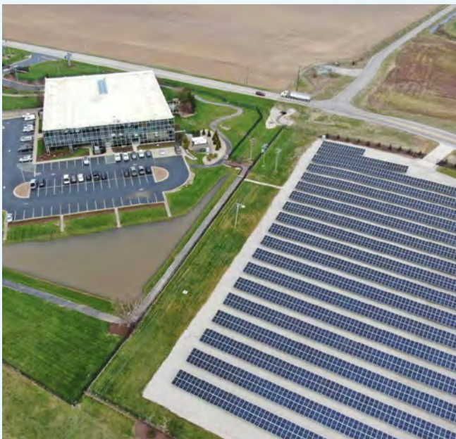
The image (above) shows Southern Star's solar field located at their HQ in Owensboro, Kentucky.
