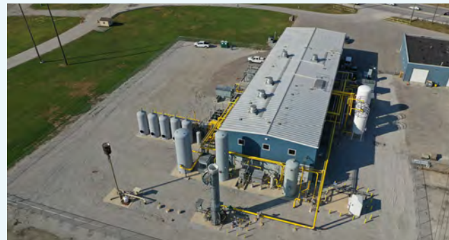
Above: Kinder Morgan's Indy High BTU facility converts landfill gas from the South Side Landfill into 800,000 MMBtu of pipeline-quality RNG each year, which when used in transport, displaces about 8 million gallons of diesel.
