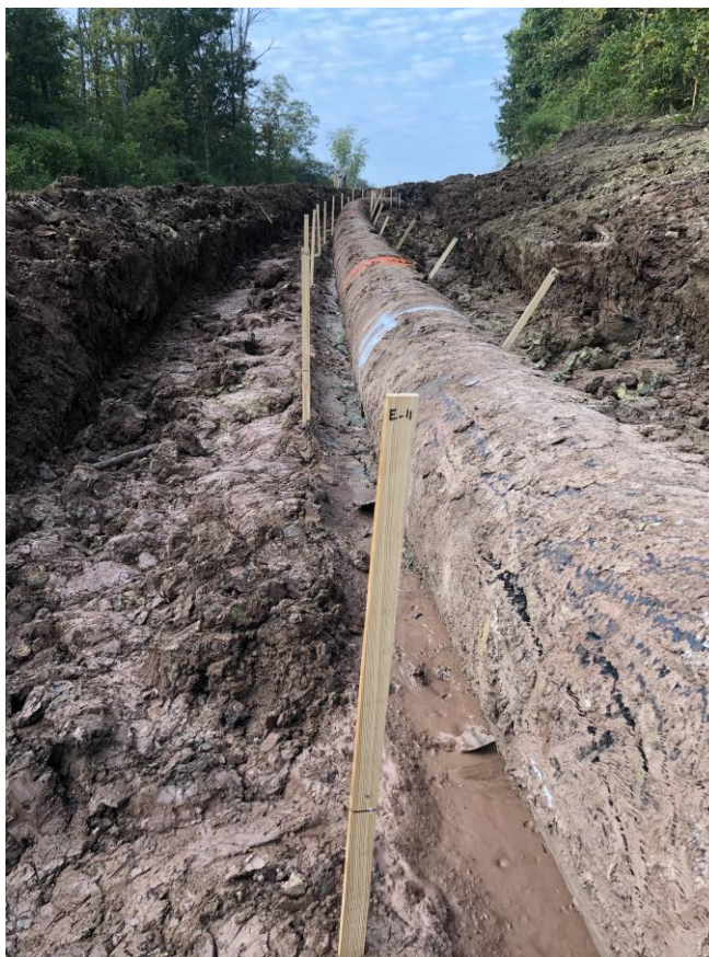
Figure G-1. Stress-relief excavation of a natural gas pipeline showing pipe rebound and survey lathes placed to provide a visual reference to measure pipe rebound
